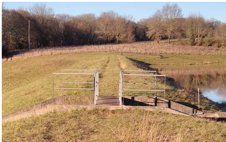
Figure 35 : Barrières garde-corps non conformes
